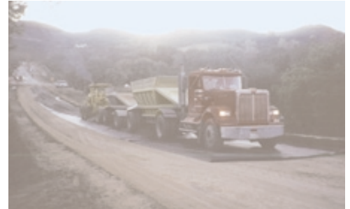
Fill was dumped and levelled over the fabric.
