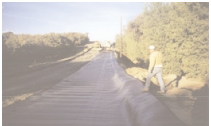
Geolon® HP570 is rolled out over the subgrade. HP570 serves two functions: to reinforce and separate.
