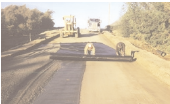
Geolon® HP570 is rolled out over the subgrade. HP570 serves two functions: to reinforce and separate.
