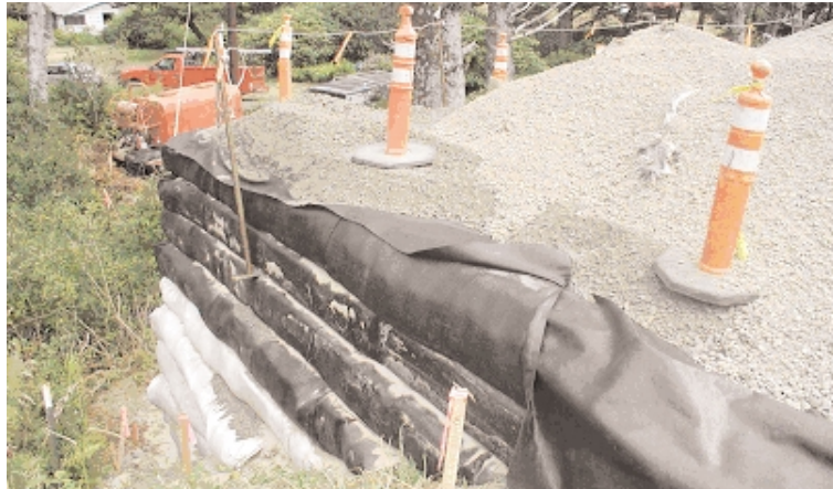
The eastern corner of the south MSE embankment.
