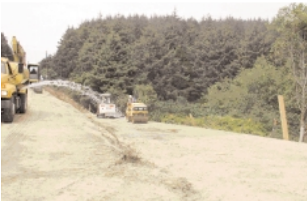
Compacting the soil before layering more Geolon® HS400.
